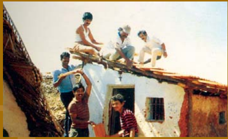
Repairing a Poor Family's House
